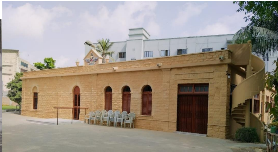
On right: newly renovated Agiary. Photo credit: Minocher Naval Vakharia
